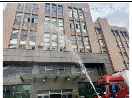
Fire hydrant testing
